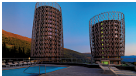
Falkensteiner edelweiss Residence
